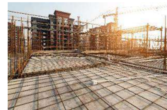
Construction steel - rebar
