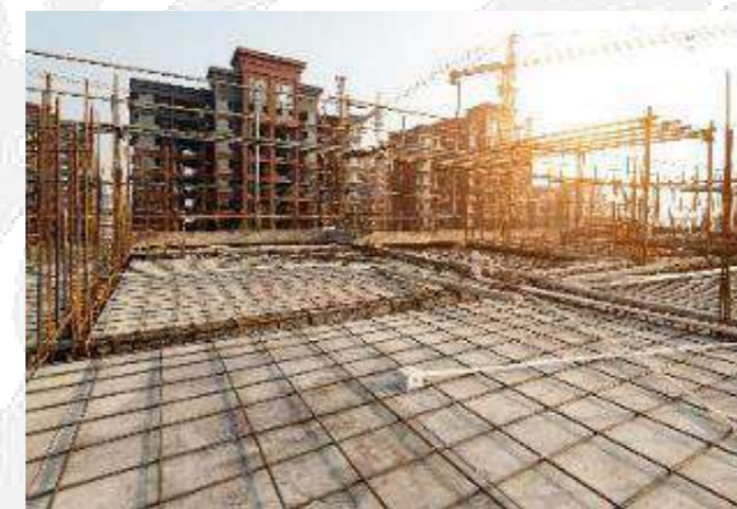
Construction steel - rebar
