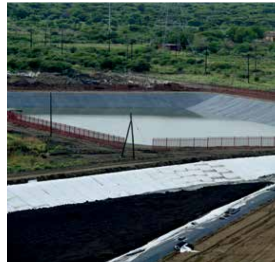
Pollution Control Dam
